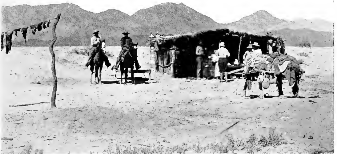
FIG. 2.—AN INDIAN HABITATION BETWEEN THE HARDY RIVER AND THE COCOPAH MOUNTAINS. THE WALLS AND ROOF OF THE STRUCTURE ARE MADE OF ARROWWEED. AT THE LEFT, A SUPPLY OF BEEF IS SUSPENDED FROM A LINE TO BE SUN-CURED OR "JERKED".
