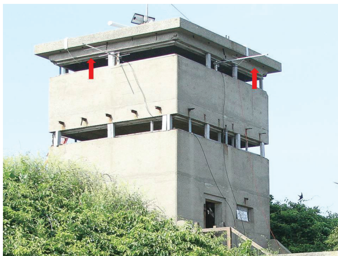
Figure 2. Observation tower on Great Gull Island where four 5-element yagi antennas (two are shown—see red arrows) were mounted as part of the automated recording station to monitor movements of Roseate Terns during the 2015 breeding season.
